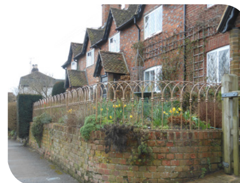
Brick wall and railings
