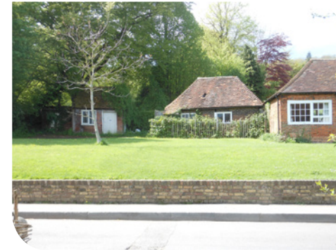
Historic ancillary buildings
