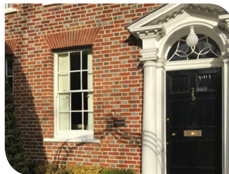
Flemish bond brickwork
