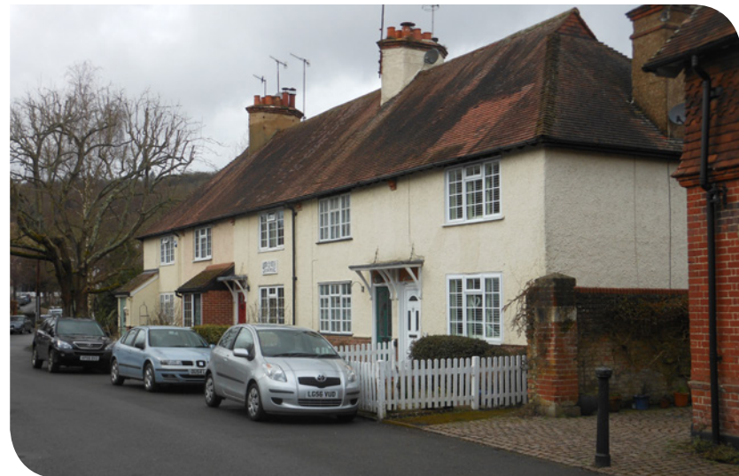
Loss of unity of a terrace of houses due to later additions
